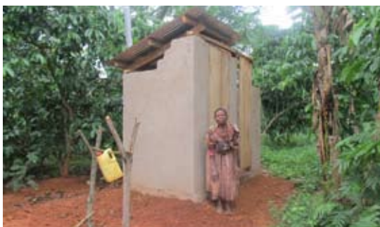
Theresa standing near her newly constructed Pit latrine With a tippy tap for hand washing
