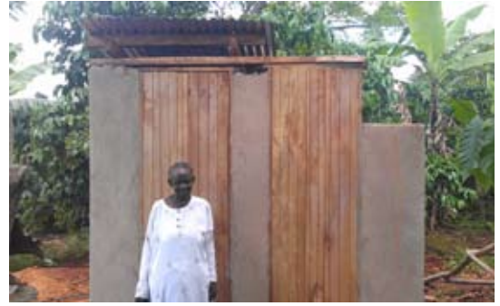
Joylance's new Latrine
