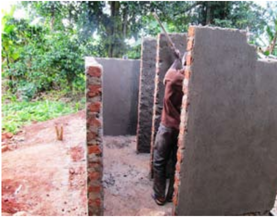
2-stance latrine and bathroom being constructed at Jjaja Margarita's home
