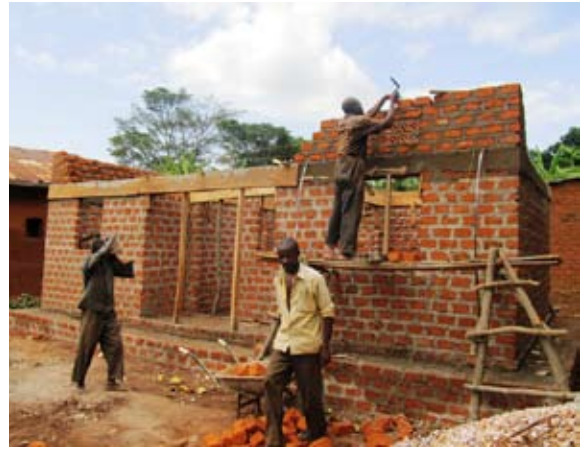
House being constructed at Jjaja Gladys's home
