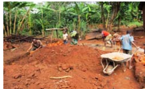
Theresa and her grandchildren actively taking part in the construction process
